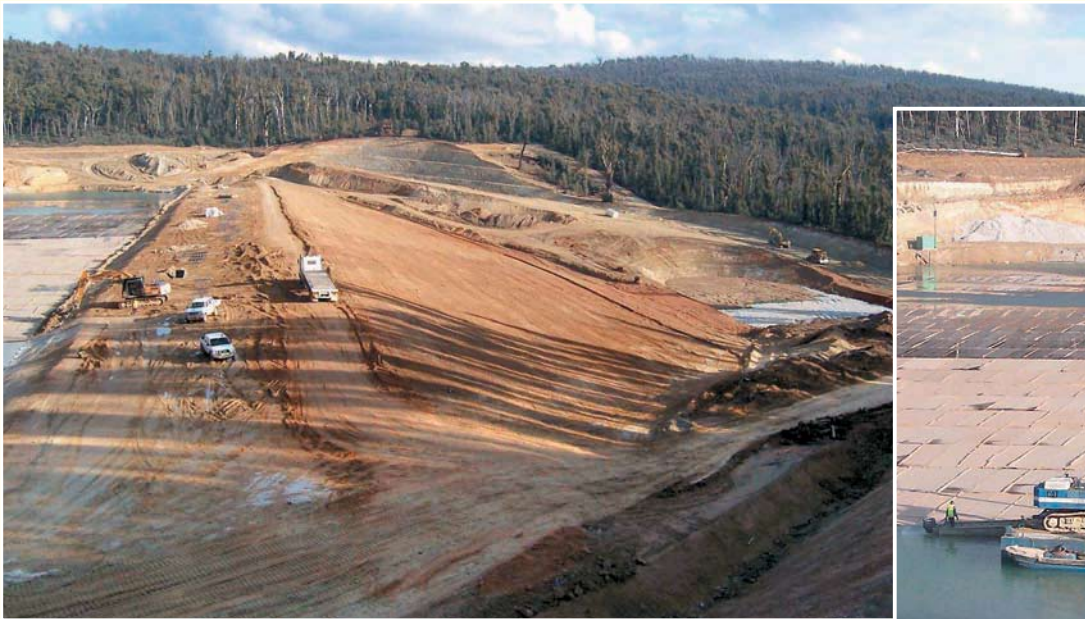
Construction of the re-engineered Tailings Dam nearing completion.
