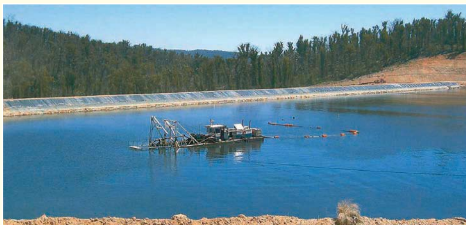
Re-levelling of the tailings with the utilisation of a dredge.
