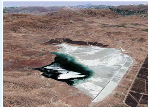
The Ovejeria storage: Presently contains 5 years of tailings production, with an estimated 50 years still to come!
