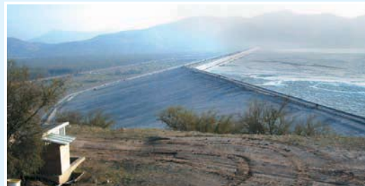
The Ovejeria embankment: The final embankment height will be significantly reduced by the introduction of a thickened tailings disposal scheme.
