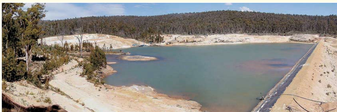
Tailings Dam site prior to rehabilitation. Note the poor distribution of the acid producing tailings.
