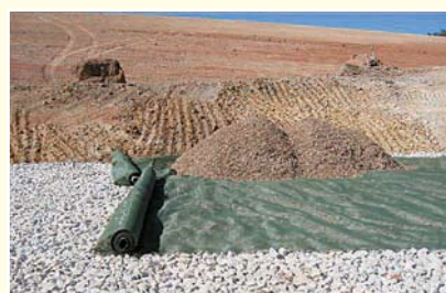
[Left] Anaerobic wetland at embankment toe under construction.
