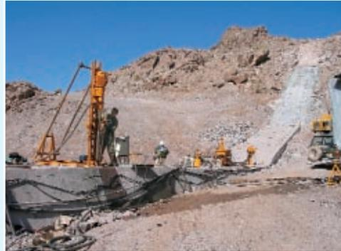
*Grouting in progress at the water retaining dam.*
