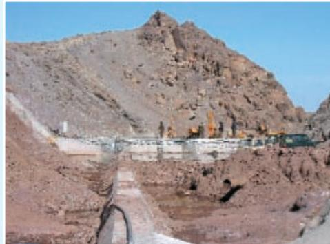
*Grouting in progress at the water retaining dam. The outlet pipe (trapezoidal concrete structure) for return water is functioning as the stream diversion.*
