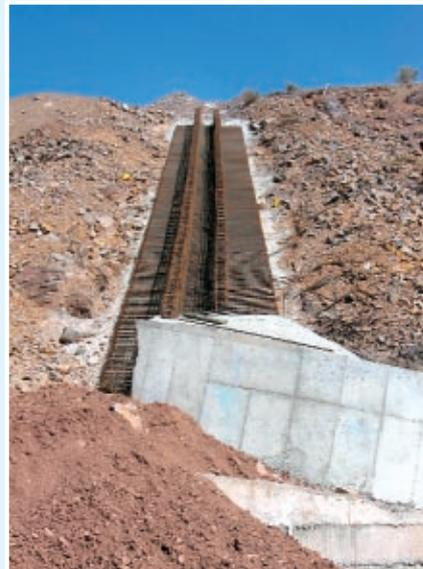
*[Right] Decant structure under construction.*
