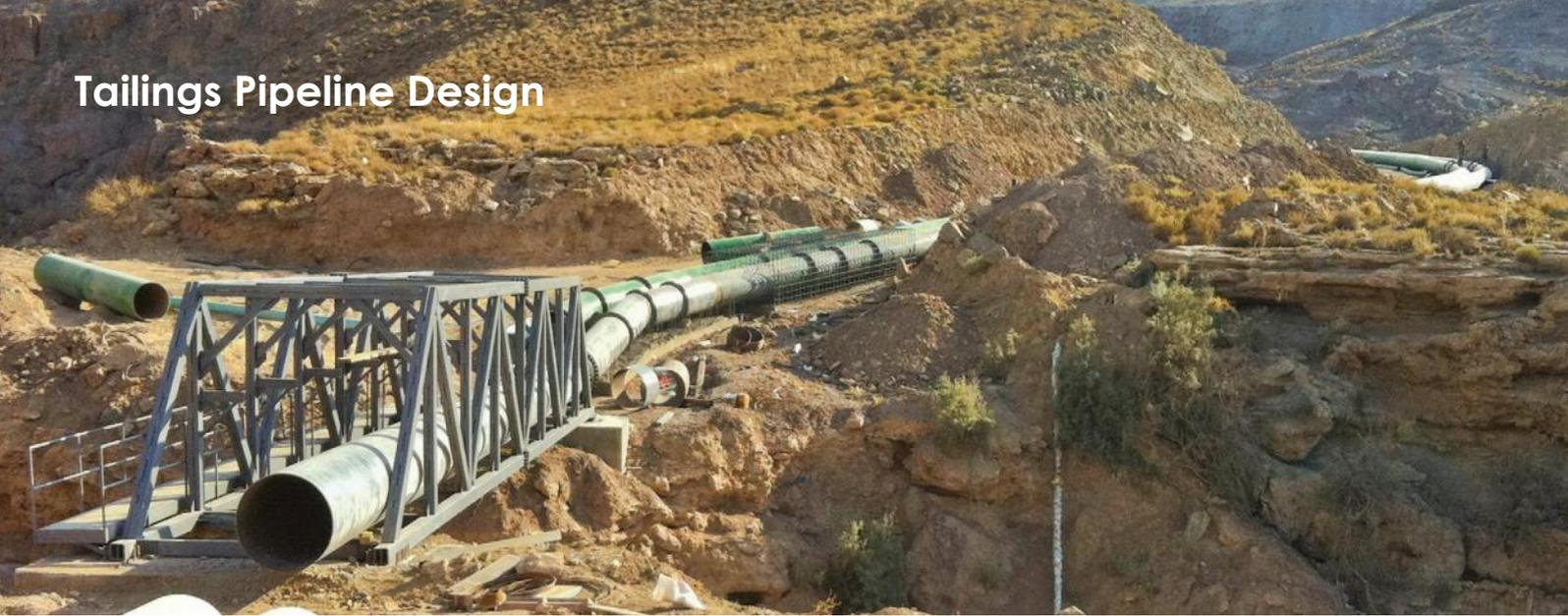
**The tailings stream from a mining operation is often in a slurry form – a mixture of solids and water – and is pumped from the processing plant to the tailings disposal area.**
